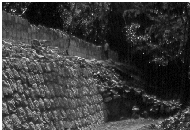
Figure 207: Terrace wall at the west side of Sacbe 1, after restoration
