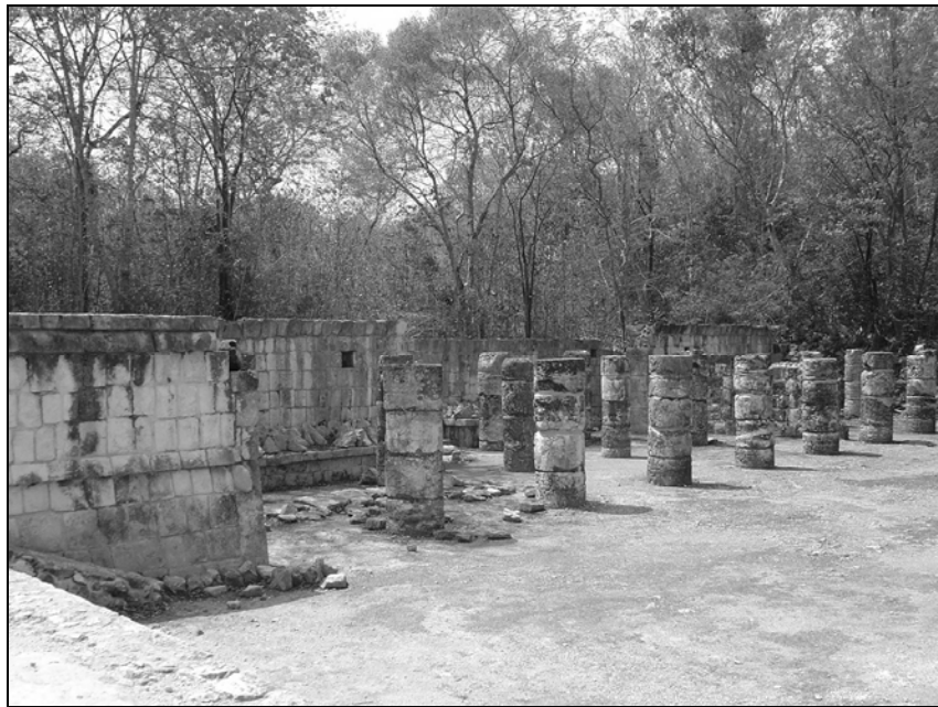
Figure 188: Structure 3D7. Frontal Gallery after clearing and restoration
