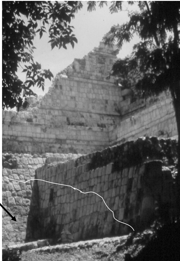
Figure 174: Location of the deposit at the back of the Northeast Colonnade
