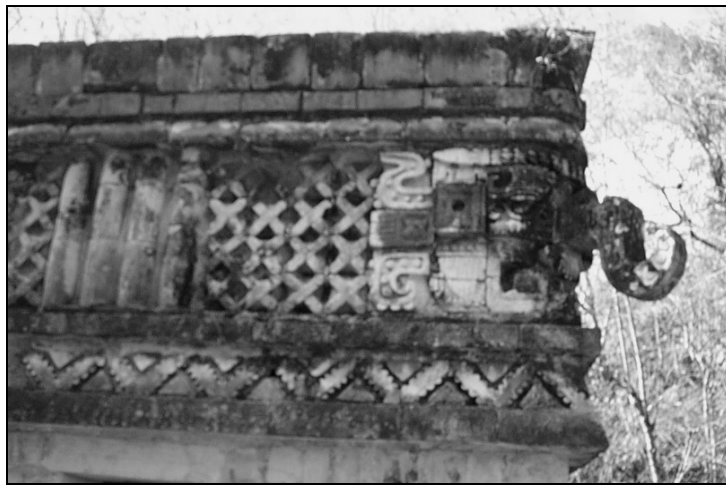
Figure 89: Frieze of the Three Lintels Building
